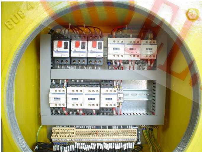
GUB - IIC control panel
